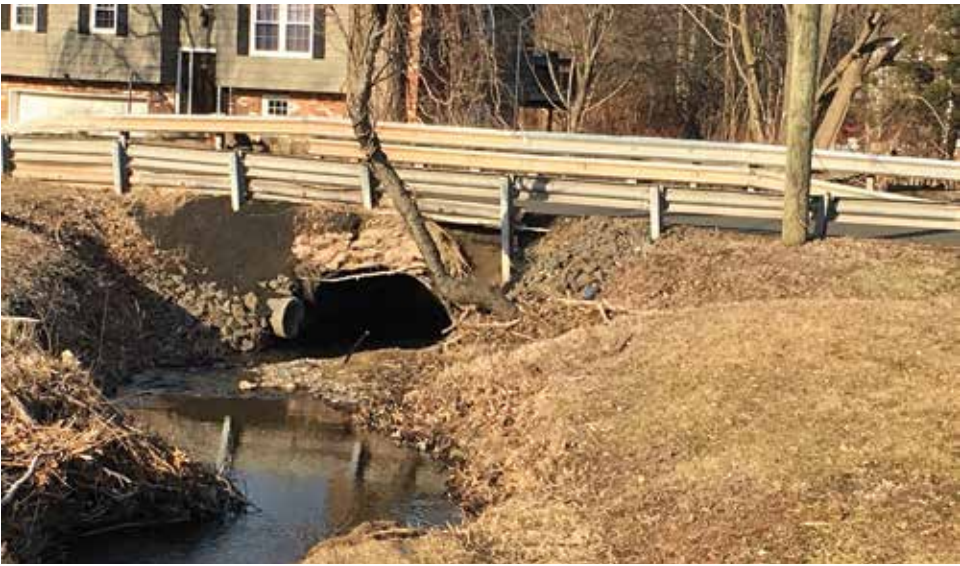
Culvert under Litchfield Turnpike contributes to flooding in major rain events.
