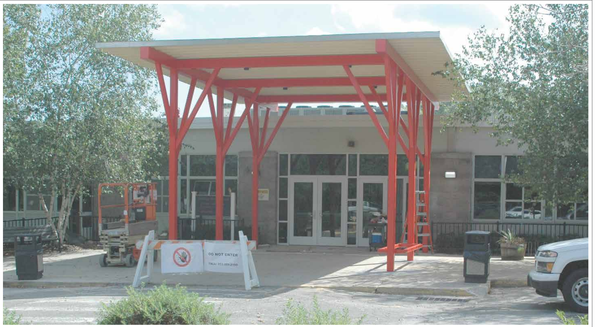
Canopies over the entrances lend Beecher Road School a new look.
