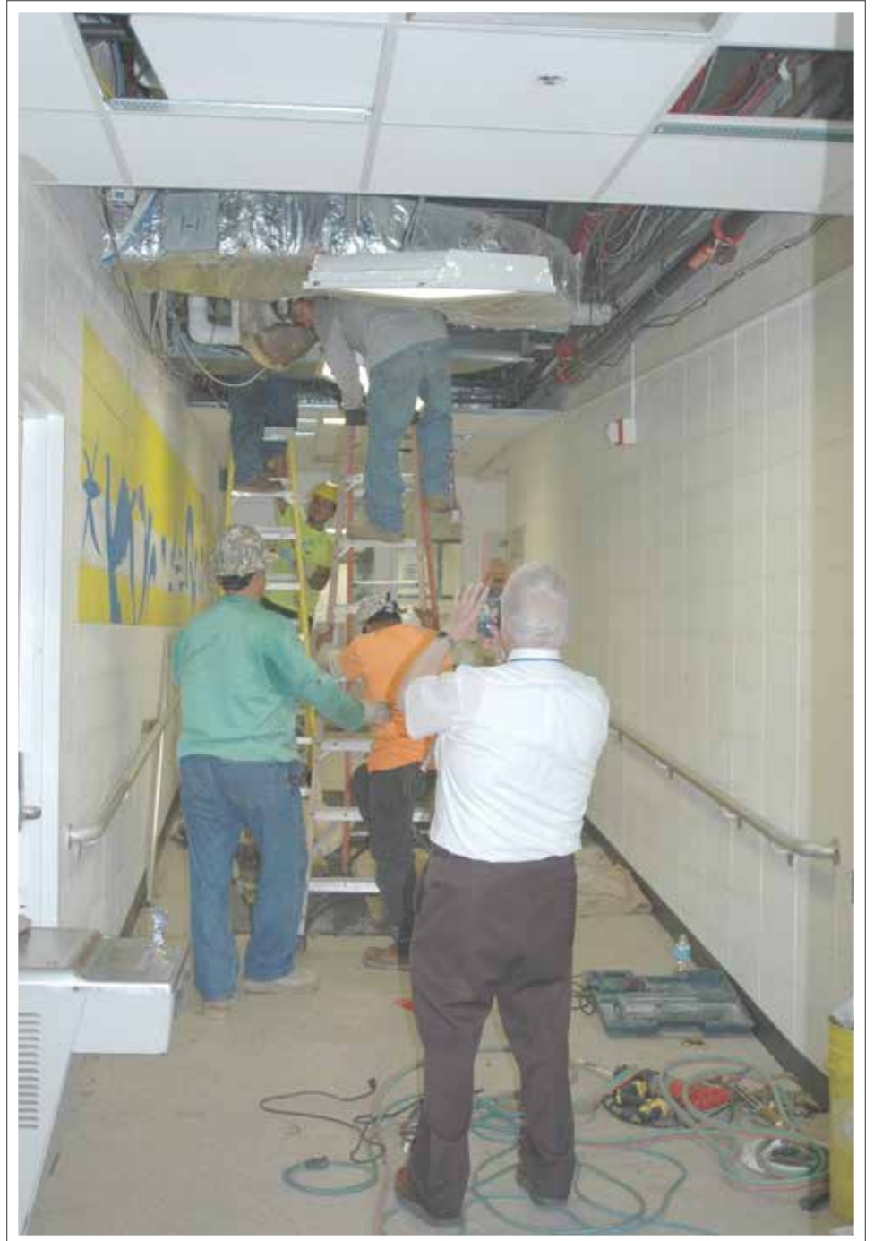
Beecher Road School was a construction zone during the summer.
