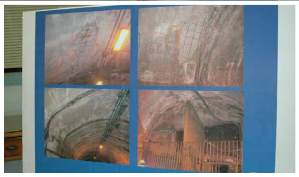
Poster showing crumbling concrete in the Heroes Tunnel.
