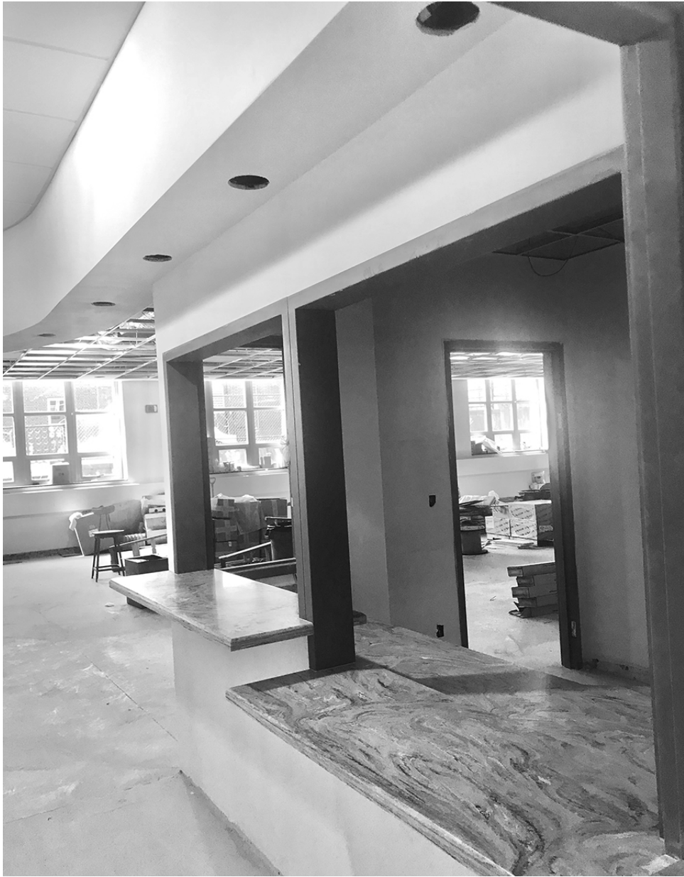
The Woodbridge Center’s renovation will be completed in just a couple of months. The Center will feature a new reception area, a consultation office, multi-use space for many programming options, and most importantly a modern and healthy ventilation system. Pictured is the new reception area. Stay tuned for information about its opening.
