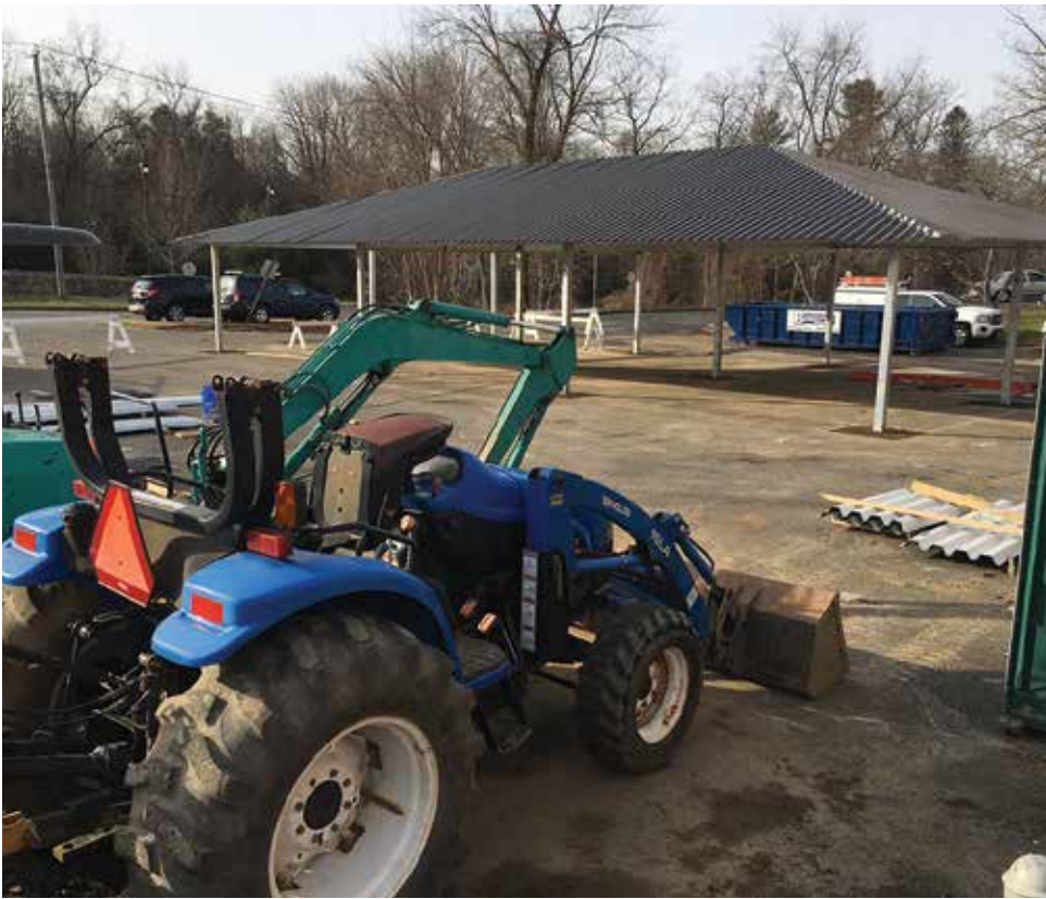
Photo of the car port being erected for the police cruisers.
